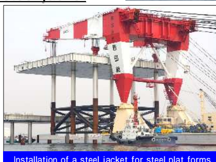
Installation of a steel jacket for steel plat forms
