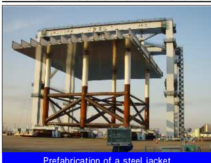
Prefabrication of a steel jacket
