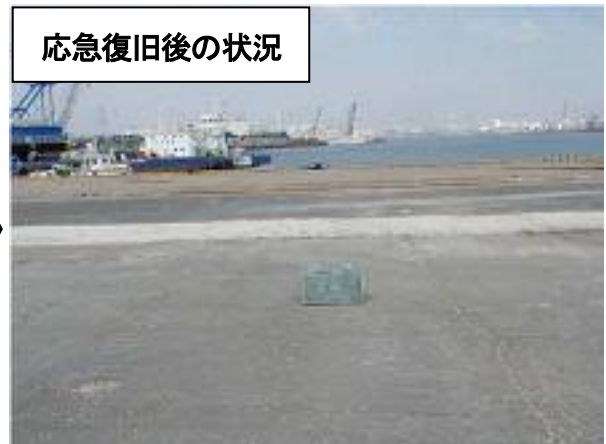
碎石を敷設し段差や陥没を解消
